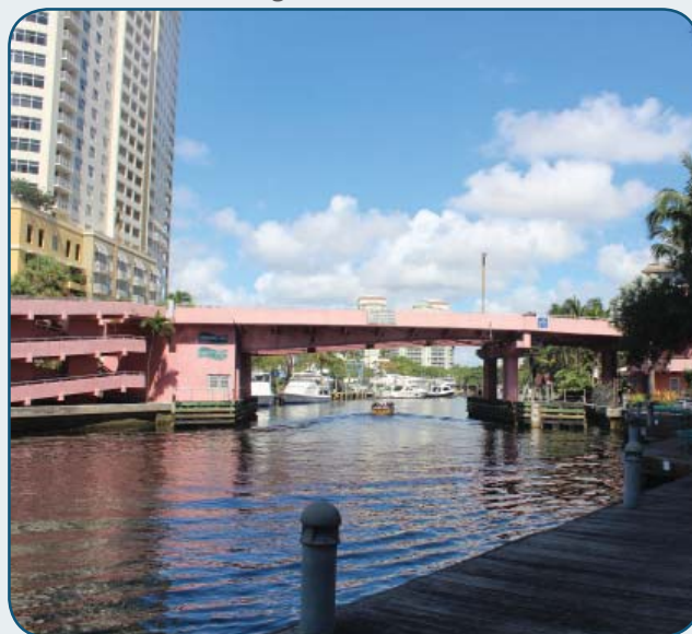
Andrews Avenue Bridge
