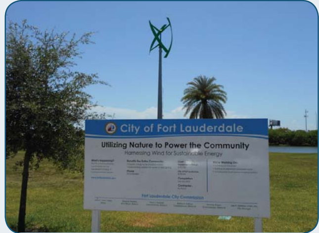
Sustainable Energy Installation at Mills Pond Park
