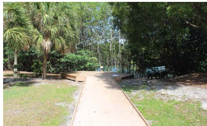
Boardwalk at North Fork Riverfront Park
